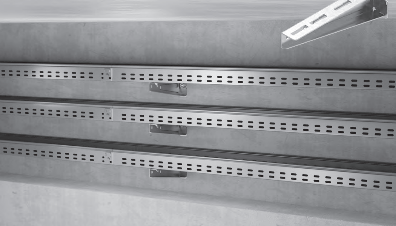
Example of multi-level route installation on new WWSR brackets...
